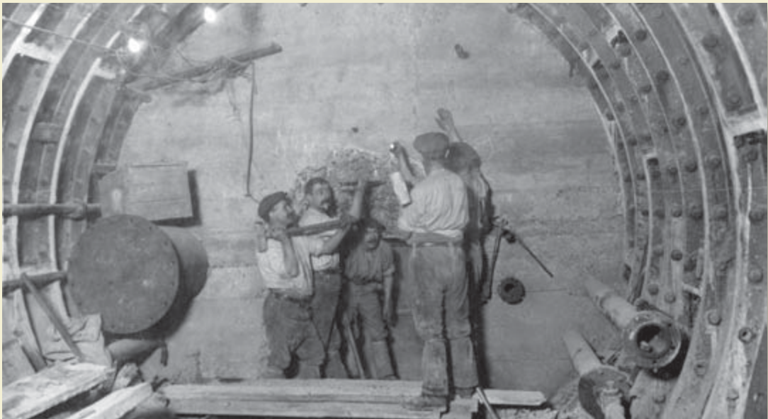
Workers removing a cement wall during expansion of the London Underground rail system in 1912. Hulton Archive/Getty Images
